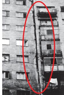
Fig. 2. Colentina district, damage down the seismic gap line, due to pounding (Pomonis et al, 1990)
