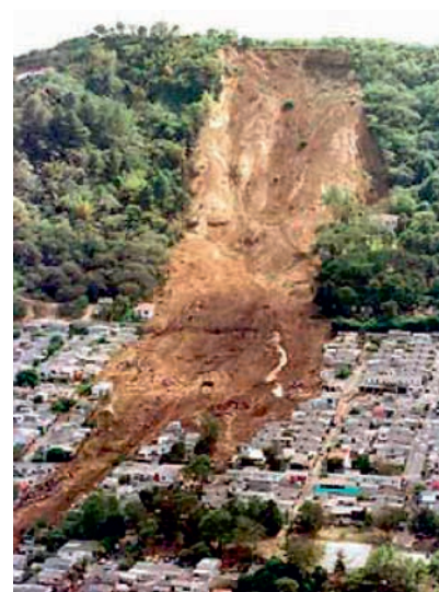
El Salvador, 2001 – alunecare de teren din cutremur ( http://en.wikipedia.org/wiki/2001_El_Salvador_earthquakes )
